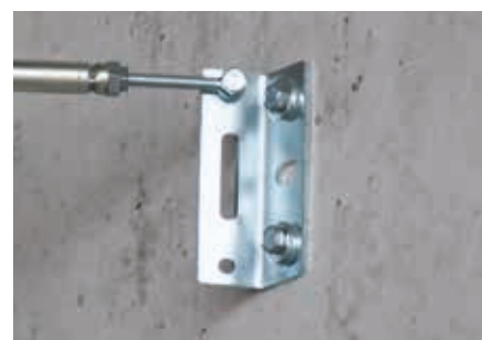
Fixing of brackets and console bearers
